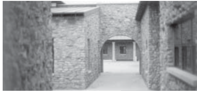
Walkway Near Courtyard
